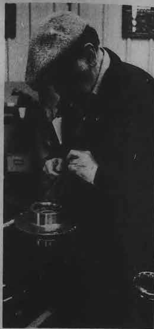
Seafarer Vincent Welch uses inside calipers to get valve measurements during a training session in the SHLSS Machine Shop. Brother Welch is attending the Pumproom course at SHLSS.
