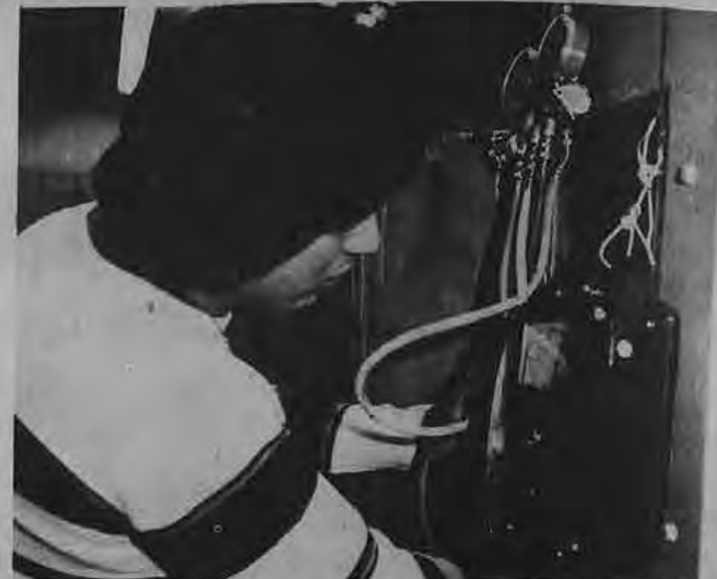
Trouble-shooting electrical systems is an important part of the responsibilities of Seafarers who are charged with the maintenance and repair of shipboard refrigeration systems. Here, Seafarer Larry Gordon runs a line check on an electrical circuit as part of his on-the-job training in the SHLSS machine shop.
