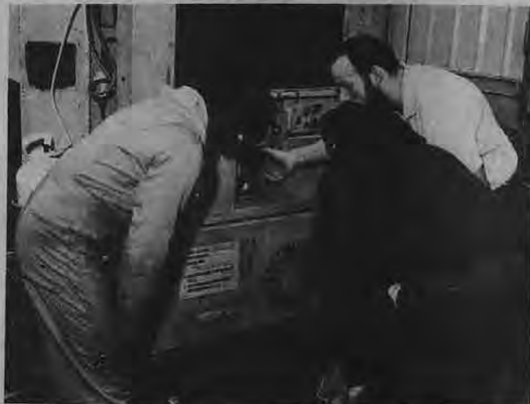
Working with the same equipment they will be responsible for aboard ship helps SIU upgraders in the learning process. Here, SHLSS instructor Eric Malzkahn explains gauge readings on a Thermo-King cooling system to two of his students.
