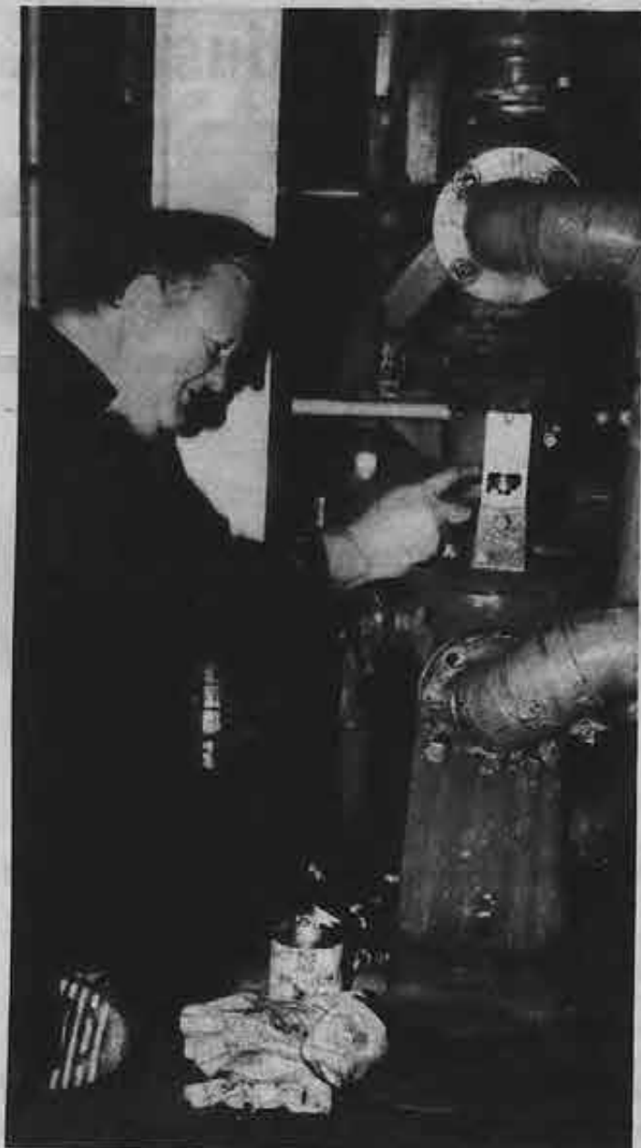
QMED Edward Elder studies where repairs are needed on the St. Clair's air-conditioning unit.
