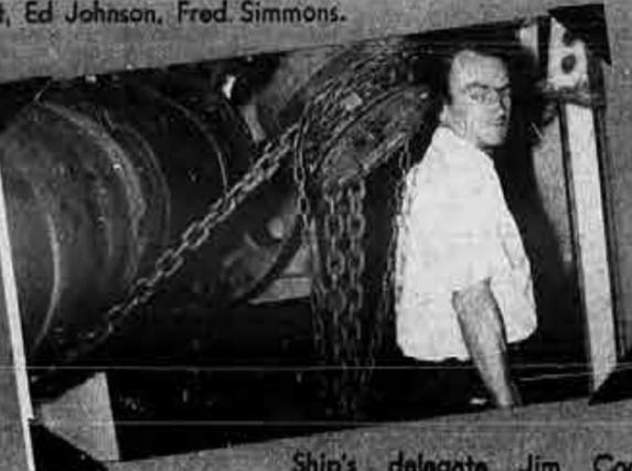
Ship's delegate Jim Cochran watches the raising of the main propulsion shaft while the Cuba Victory was undergoing repair work.
