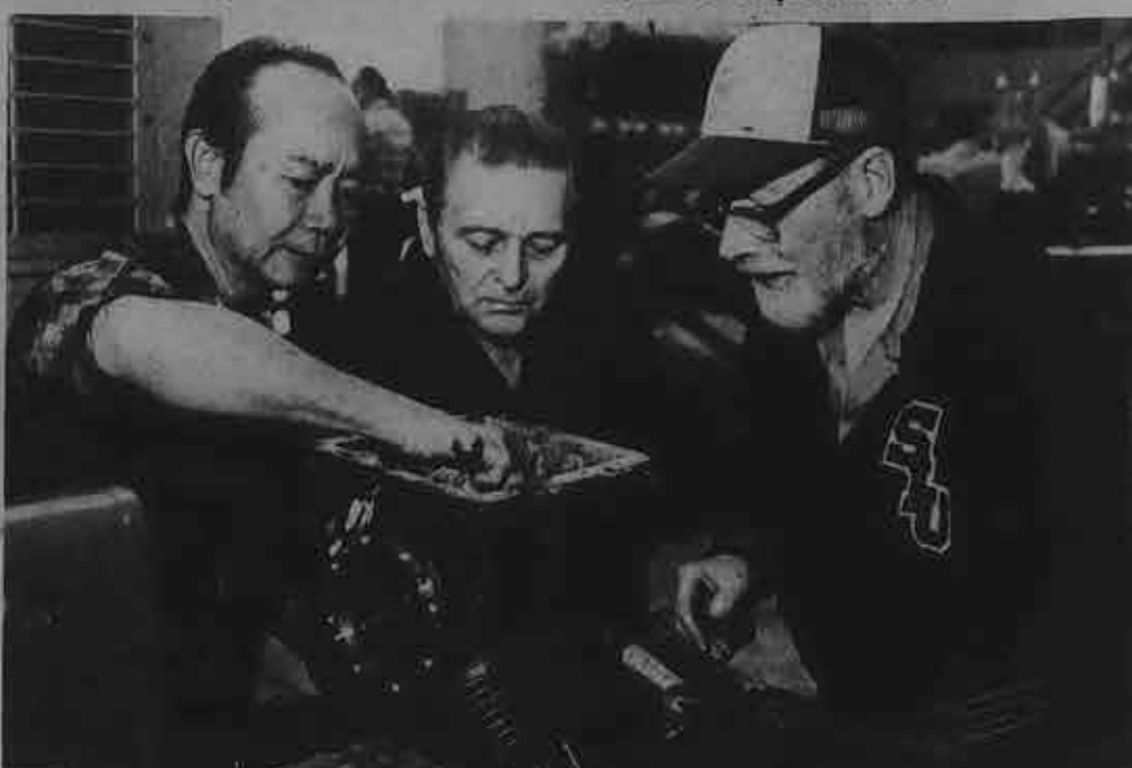
Hands-on training is an integral part of all of the upgrading programs at the Seafarers Harry Lundeborg School of Seamanship and the course in refrigeration Systems is no exception. Here, three Seafarers from widely separate areas of the U.S. work together to repair a compressor. From left are Exequiel Liwag, Port of Norfolk; William Katt, Port of Chicago, and Louie Guertin, Port of New Orleans.
