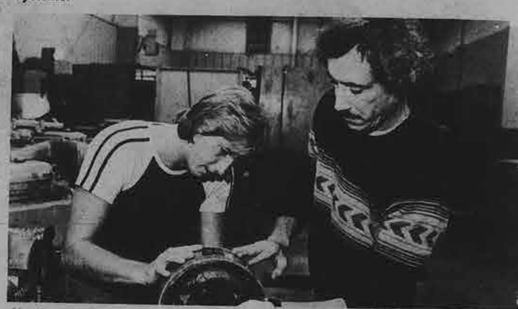
Hands-on experience is very important in all of the upgrading programs at SHLSS. Here, Seafarers Jim Pyle, from the Port of Tampa, and Dave Morgan, Baltimore, do some troubleshooting on an electric motor as part of their course in Marine Electrical Maintenance.
