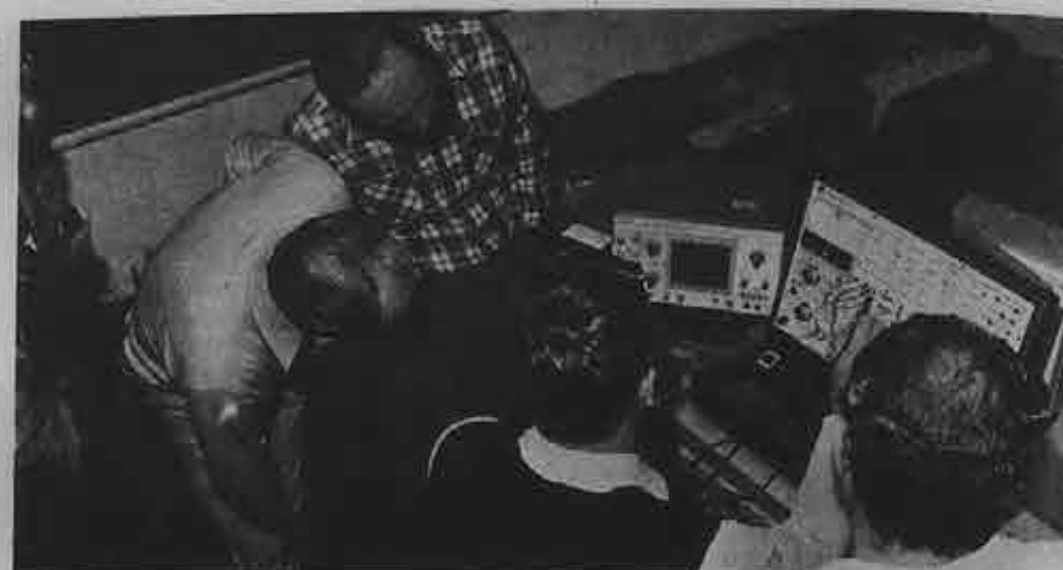
The practical instruction is given on desk top pieces of equipment, oscilloscopes and oscillators. Seafarers can make a circuit and test it during their training.
