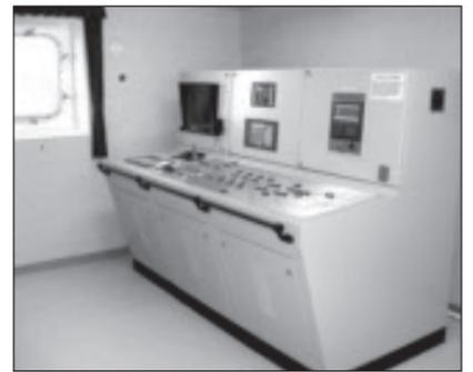
This is a ballast water control console aboard the *Horizon Hawk*.
