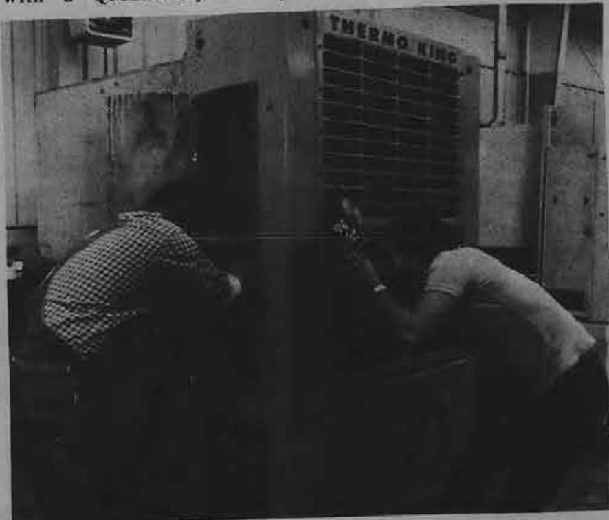
Checking the high and low side pressures with a manifold gauge is demonstrated by Dan Doyle of New York, and Bill Gizzo of Wilmington.
