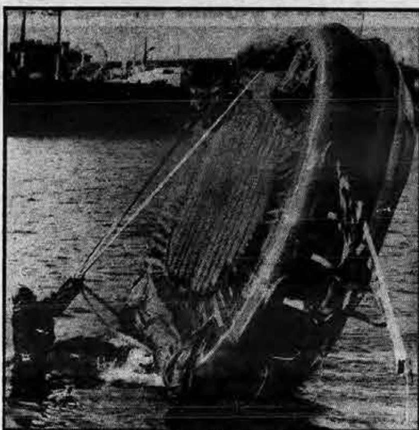
Now accepted by Coast Guard for use on American-flag ships, self-inflating life raft is shown during demonstration. Here it is being righted after landing upside down. Rafts can supplement lifeboats on ocean-going ships.
