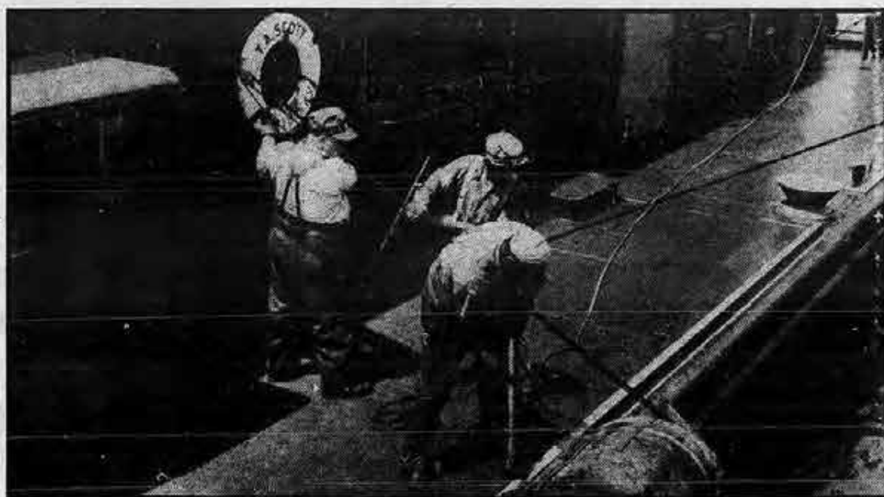
Putting scowbumper on SIU-affiliated diesel electric dipper dredge T. A. Scott (Merritt, Chapman & Scott) are (l-r) Leonard Thornton, operator, and Frederick Robear and Tom Nault, deckhands. Bumper protects dredge from being damaged while it is loading scow.
