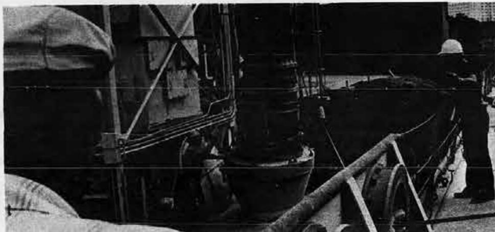
The cement pours through this boom and its telescoped end.
