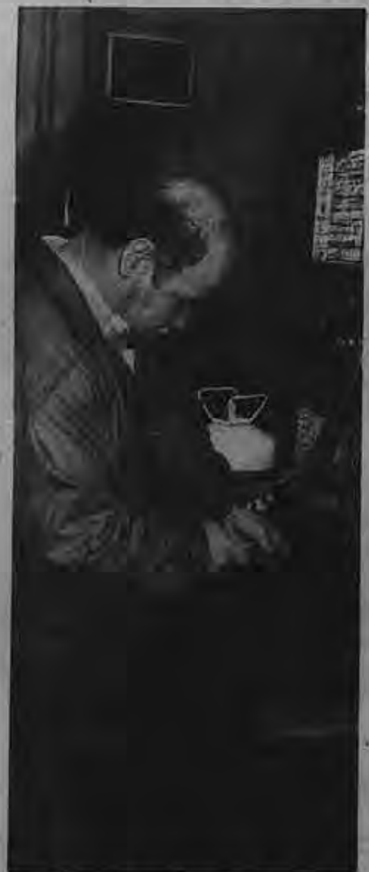
Seafarer Bob Benson, from the Port of Seattle, works on the coolant system on a working mock-up of a typical refrigeration system.
