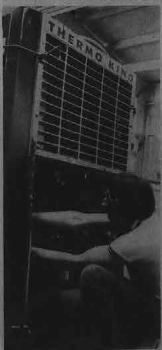
Seafarer Edward Marks of Seattle learns maintenance procedures on the coolant system of reefer boxes as a part of the QMED upgrading program at SHLSS.
