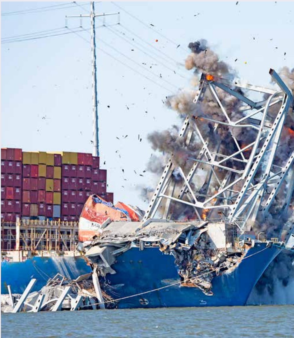
Salvors with the Unified Command perform a controlled demolition and precision cutting of a section of the Francis Scott Key Bridge that sits on the port side of the bow of the Dali in May 2024. (Photo by USACE public affairs specialist Elizabeth Lockyear)
