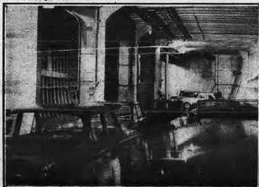
SPACIOUS INTERIOR hold is used for "roll-on" cargo such as autos, as well as additional trailer bodies brought in by fork-lift.
